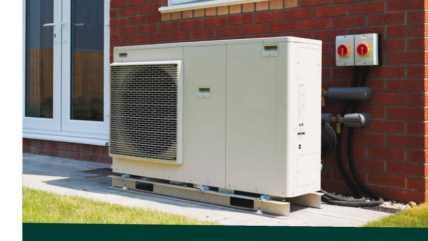
Your ASHP will normally be located under the window of the rear elevation, and the hot water cylinder will be located in a first floor cupboard. The cylinder will be between 150 and 300L in capacity, depending on the size of your home. Refer to your floorplans for the exact position in your house type.
